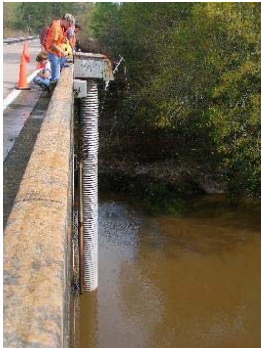
Figure 26 USGS continuous monitoring station at site E1
