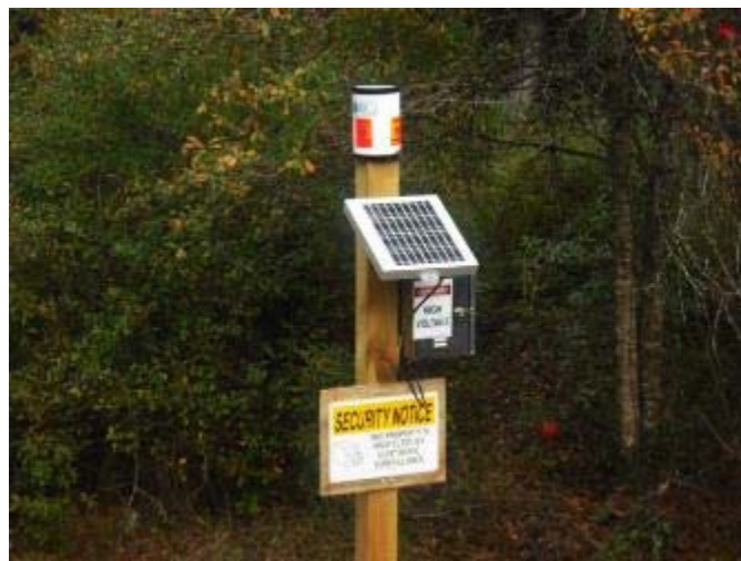
Figure 24 Continuous real-time monitoring station installed at site B6
